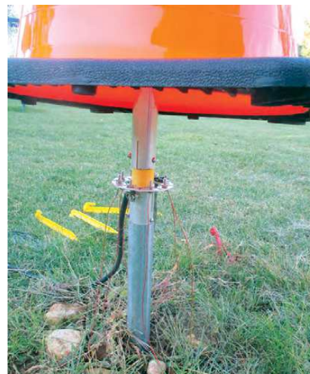
Figure 3 — The traffic cone over the open connections on the lower part of the antenna. [Robert W. Lobenstein, WA2AXZ/9, photo]
