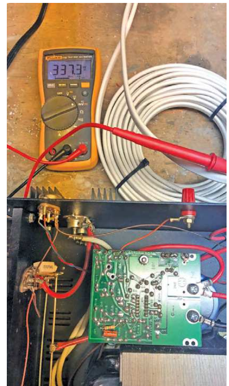
Figure 5 — I connected my digital multimeter to the short segment of dummy load wire and was able to read the current and calibrate the ammeter. [Steve Masticola, WX2S, photo]
