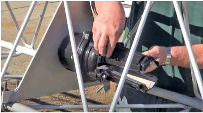
As part of Randy's, K7AGE, tower installation series, he demonstrates how to mount the rotor to the tower.
