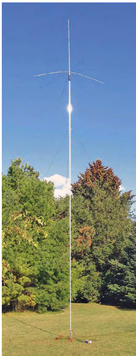
Figure 1 — The Cushcraft MA-160V antenna in my yard, before I buried the radials. [Robert W. Lobenstein, WA2AXZ/9, photo]
