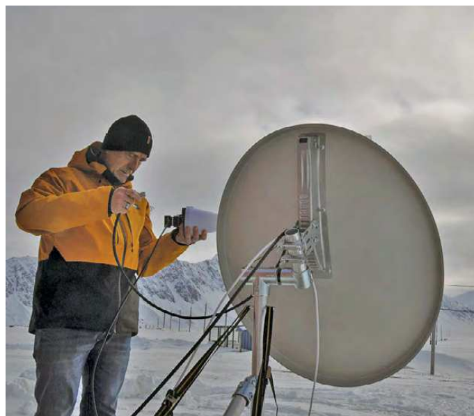
Patrick Blancquaert, ON4DCU, during the installation of the Triax satellite antennas. The team brought two 120-centimeter antennas because they were active with two stations at the same time on the QO-100 satellite.
