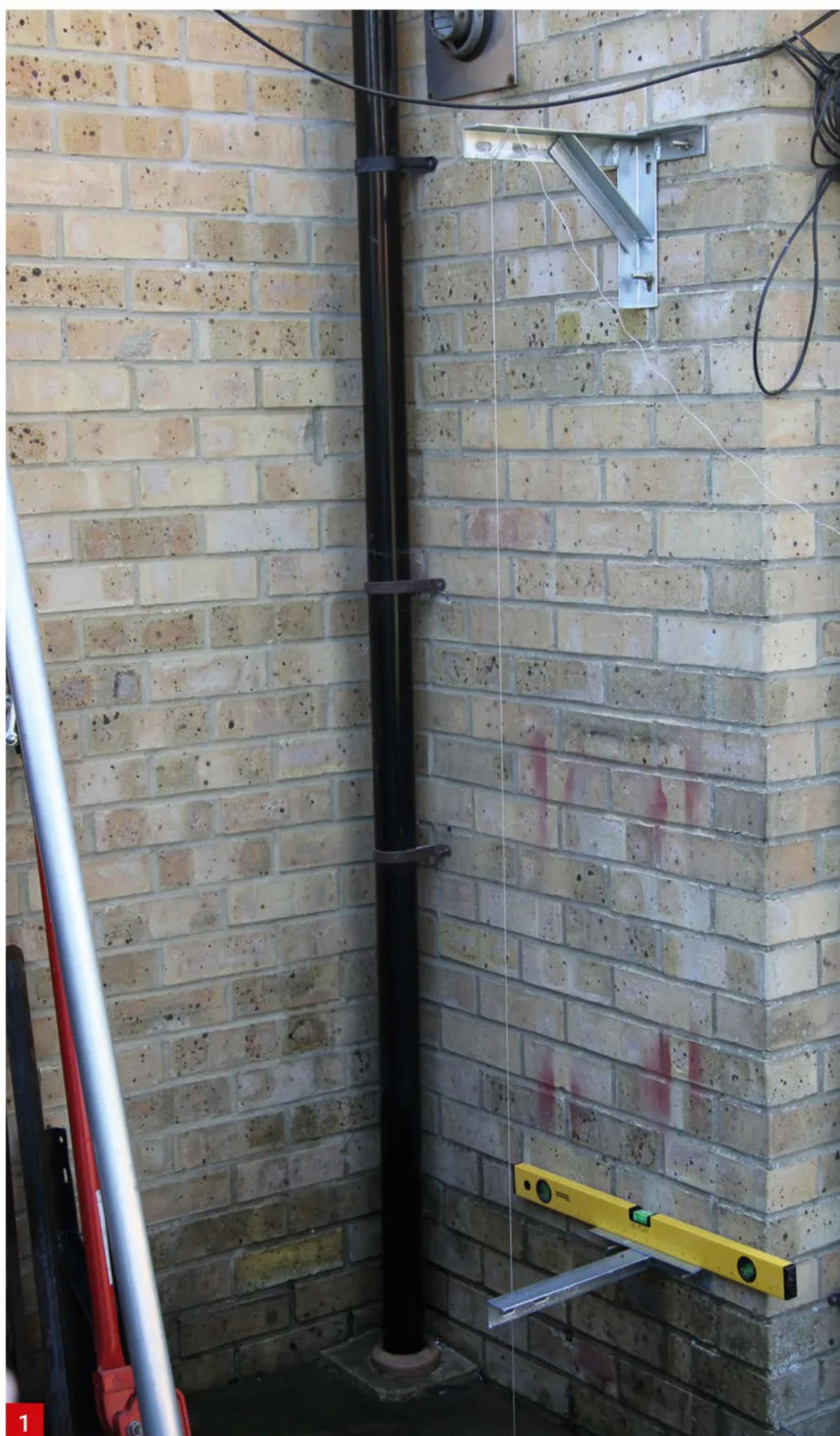
Fig. 1: Brackets being installed. Note the proximity of the lower bracket to the DPC.
