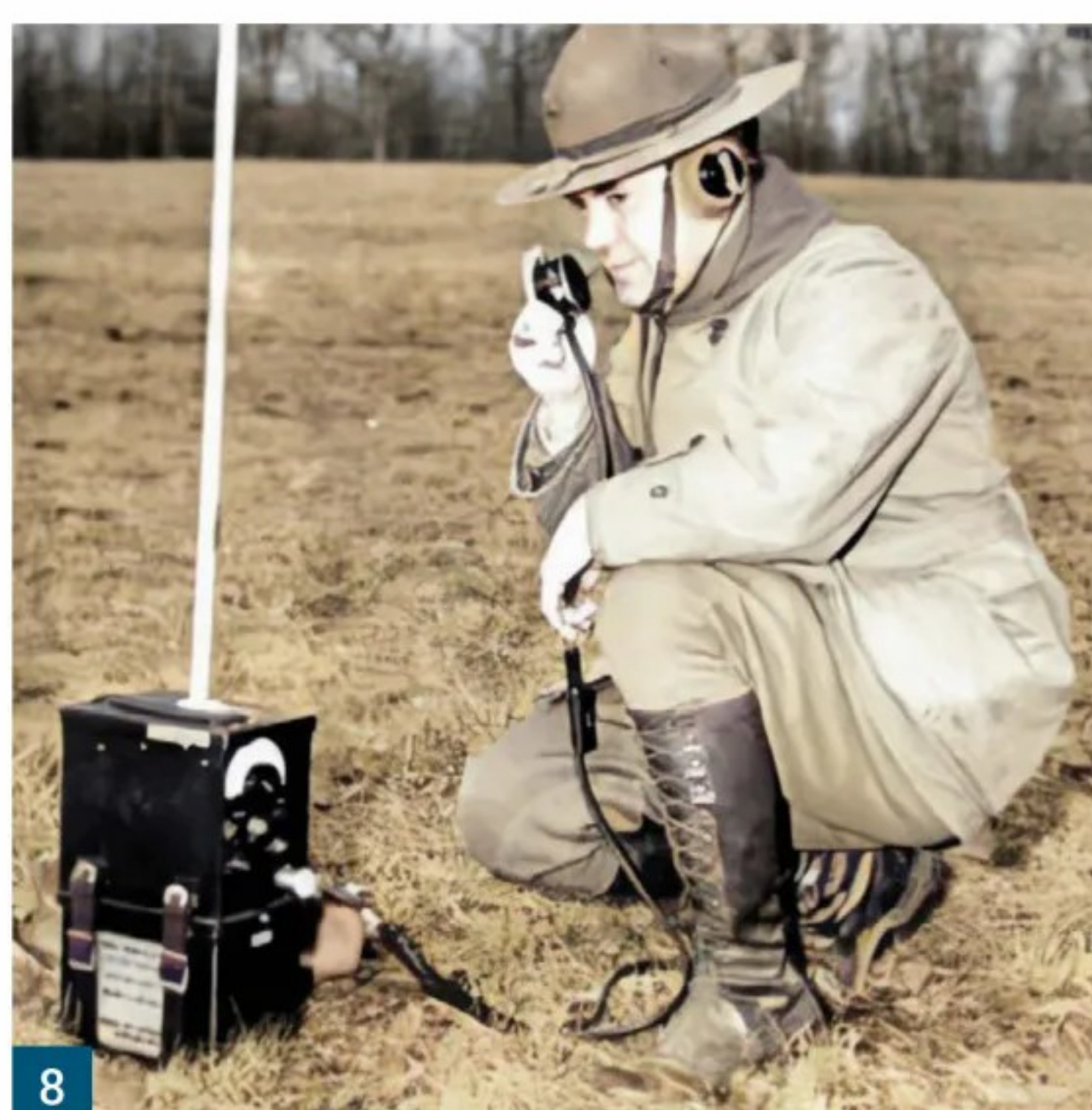
Fig. 3: The 30.7 x 30.1 x 18.4cm TBV's aluminium cabinet housed the transceiver and dry battery pack. Carried in a canvas case, together with the sectional antenna, the man-pack weighed 15.2kg. ( invaluable.com ) Fig. 4: A US Marine Navajo Code Talker operating his TBV radio. The Japanese were never able to understand their language, which proved to be more successful than using standard code. Fig. 5: The BC-322 transmitter-receiver for the lightweight SCR-195 radio is carried on the back of the operator in a canvas bag, together with the telescoping tubular antenna and battery, for a total weight of only 12.15kg. ( armyradio.ch ) Fig. 6: The lightweight SCR-195 portable company-battalion level radio, which had a range of up to five miles, is seen here inside its canvas backpack. ( imageevent.com ) Fig. 7: Left: the SCR-194 artillery observer version. Right: the SCR-195 infantry version. Also illustrated are the radio's backpacks, base for the antenna, TS-11 headset and box BX-13 for added connection ports. ( Radio-us-ww2.blog4ever.com ) Fig. 8: This pre-war publicity photograph illustrates the SCR-194 operated as a ground station. The operator is using a T-24 microphone and is wearing the TS-11 headset. ( timetoast.com ) Fig. 9: This photograph provides a clear understanding of how the lightweight SCR-195, when carried in a backpack, can be operated by one man on the move. ( life.com )
